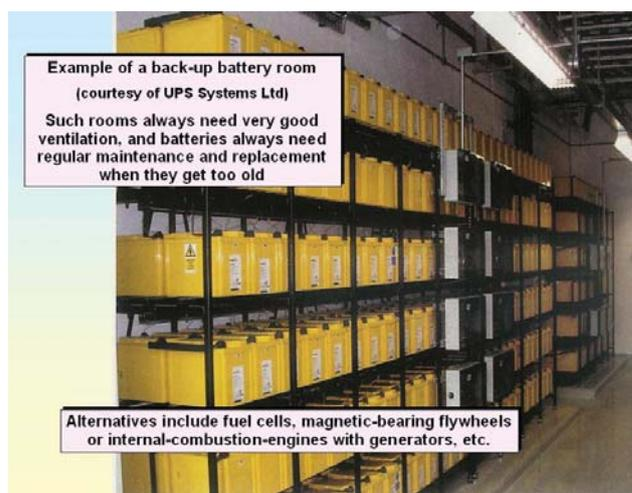
Figure 6BK Example of a large battery room
