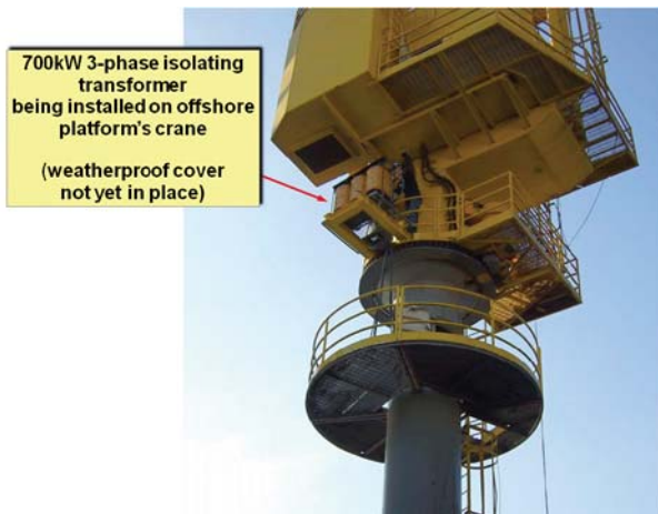
Figure 5.2-3 The fix for the CM noise from the crane motor drives
